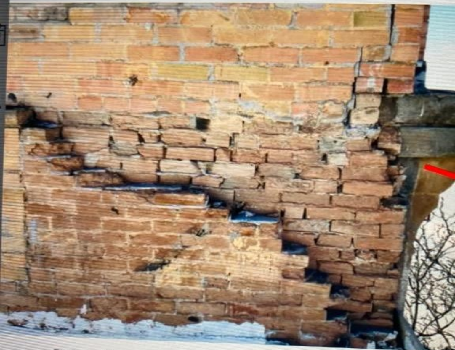
Northeast corner bricks
