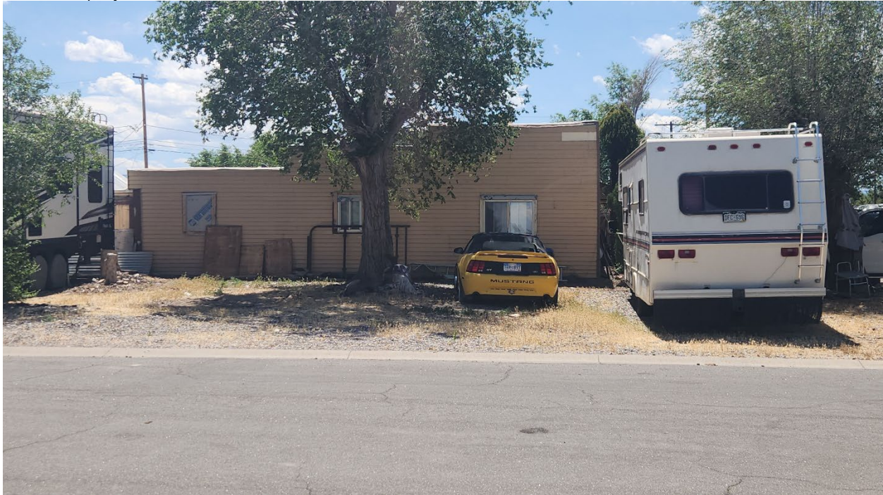
Photo 11 Northwestern façade of 1930 WPA modernist building including low-slope roof behind a stepped parapet at 540 North Ute Avenue (site 5MN13355), camera facing southeast
