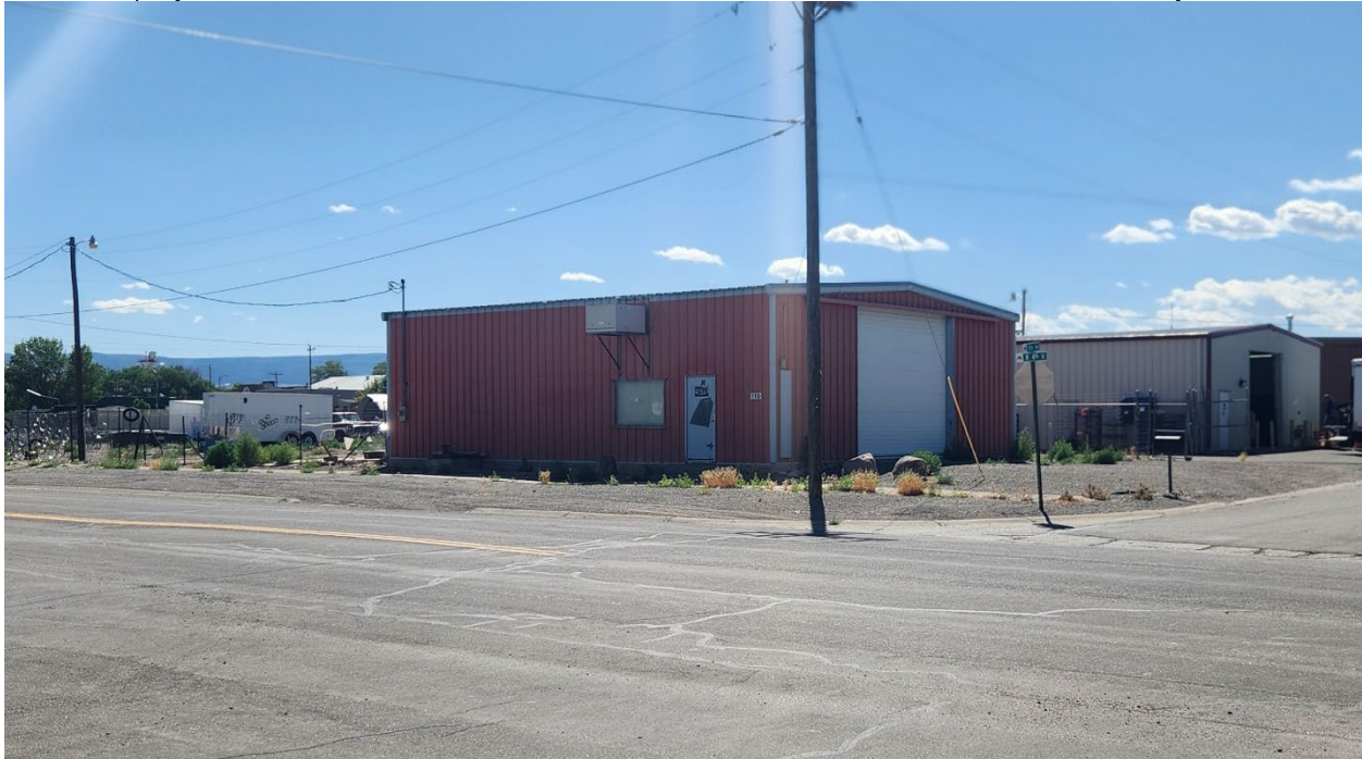
Photo 17 Western side of 1967 steel-framed warehouse at 110 North Fourth St. (site 5MN12944), camera facing east
