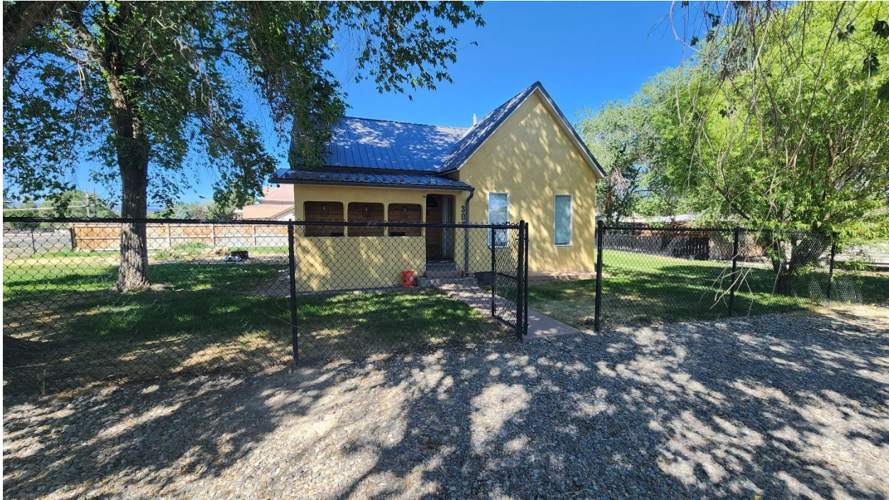
Photo 1 Northeastern (main) façade of 1900 gabled vernacular with stucco finish at 305 North Ute Ave (site 5MN13409), camera facing southwest
