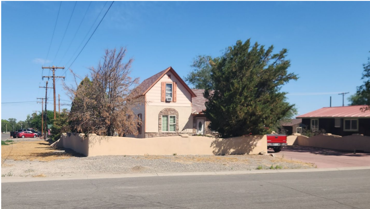
Photo 2 Southeastern side of a 1900 two-story gabled vernacular with partial stucco finish at 129 North Seventh St. (site 5MN13414), camera facing northwest
