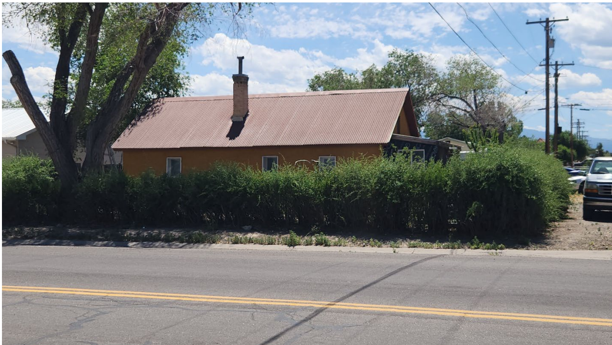
Photo 8 Northwestern side of a 1922 masonry vernacular building with stucco finish at 840 North Ute Avenue (site 5MN13360), camera facing southeast
