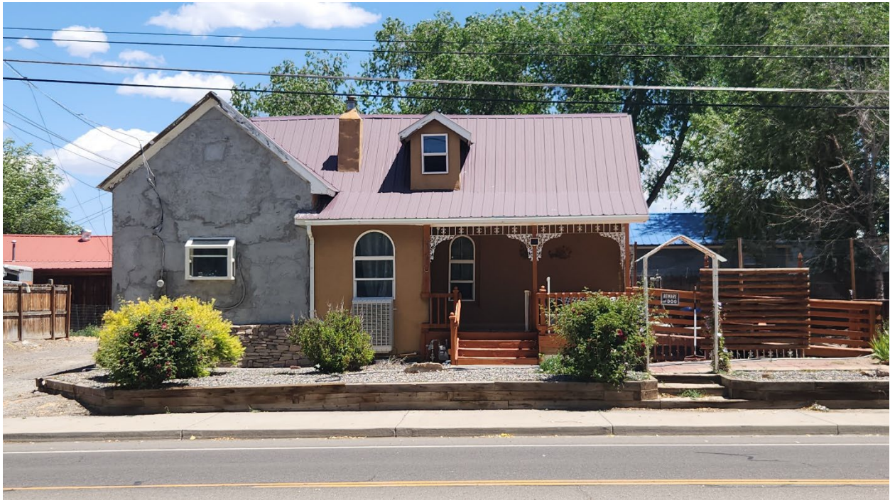
Photo 3 Southwestern façade of 1880 gabled vernacular with stucco finish at 420 North Grand Ave (site 5MN13408), camera facing northeast
