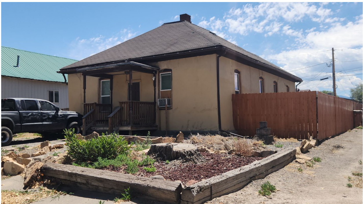
Photo 4 Northwestern side of 1910 vernacular masonry cottage with stucco finish at 340 North Grand Ave (site 5MN13368), camera facing southeast
