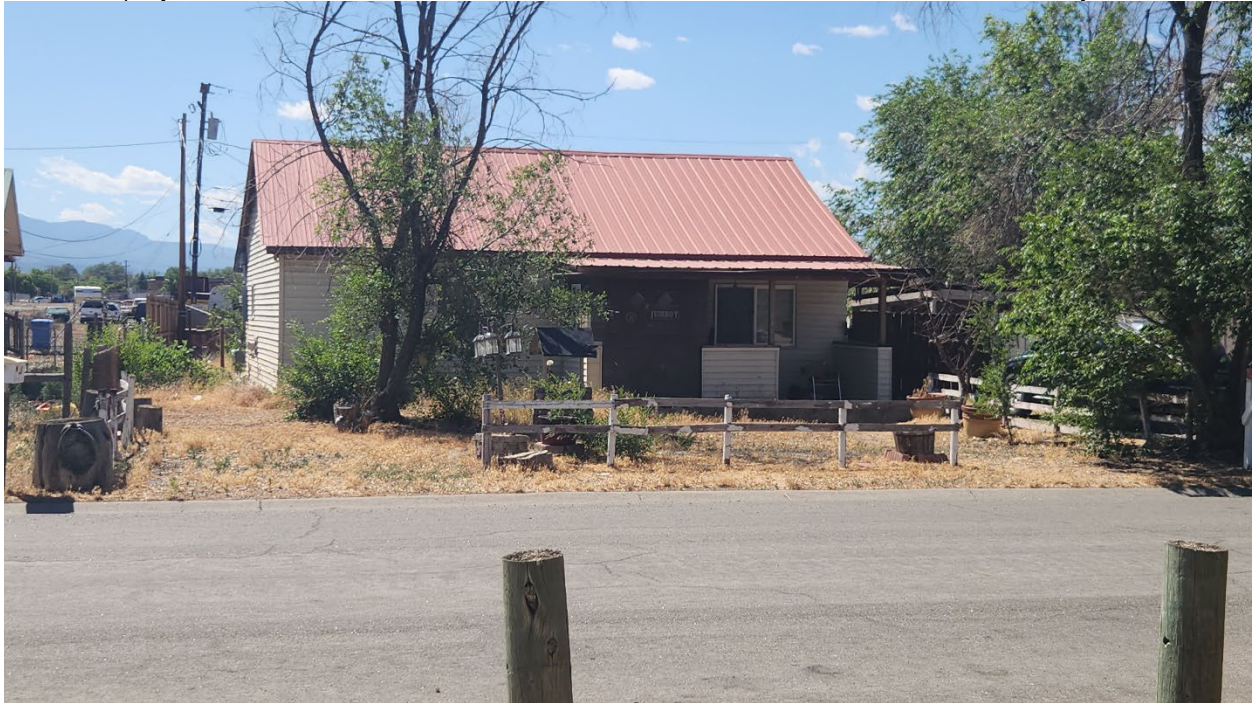
Photo 13 Northwestern side of 1948 gabled vernacular linear plan masonry building at 146 North Sixth St. (site 5MN13381), camera facing southeast
