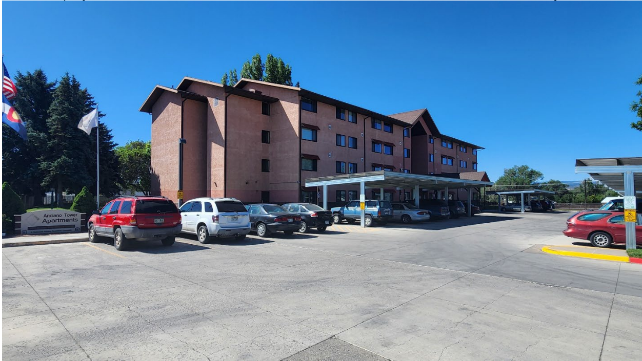
Photo 21 Northern side of 1985 Anciano Towers with stucco exterior, camera facing south
