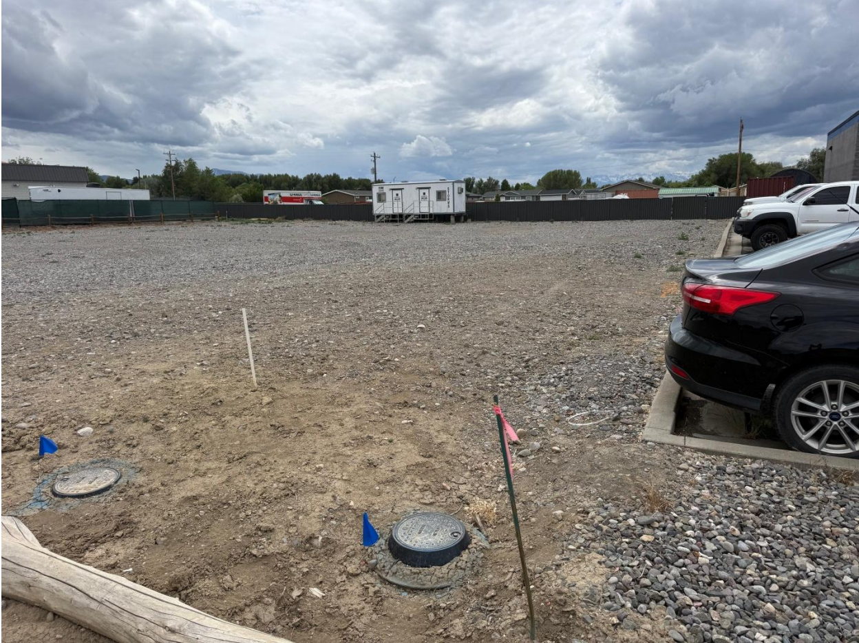
Photo 1 – View from northwest property corner looking south east.
