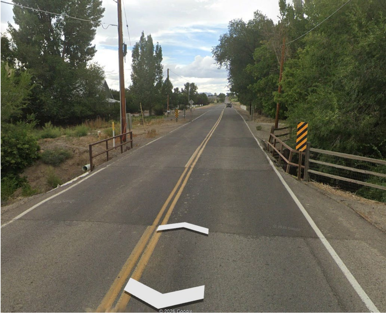
Photo 1: Existing 6700-Cedar Creek Bridge
