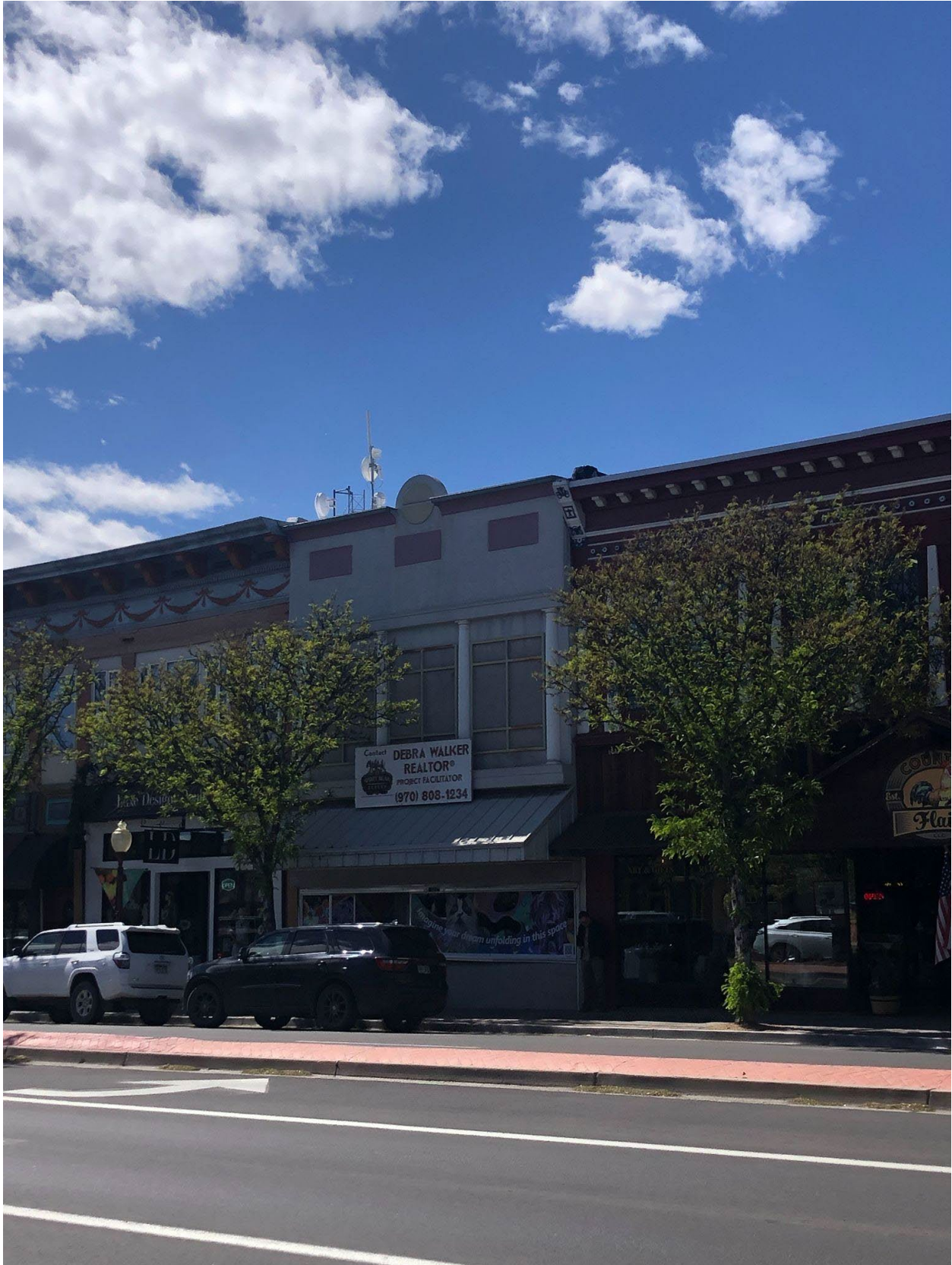
Front Facade. Second story is divided by classical columns. Between the columns are paired three-part windows.
