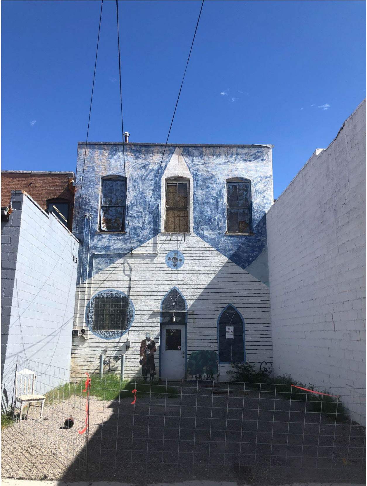
Building rear. Second story windows feature arched lintels and stone sills.
