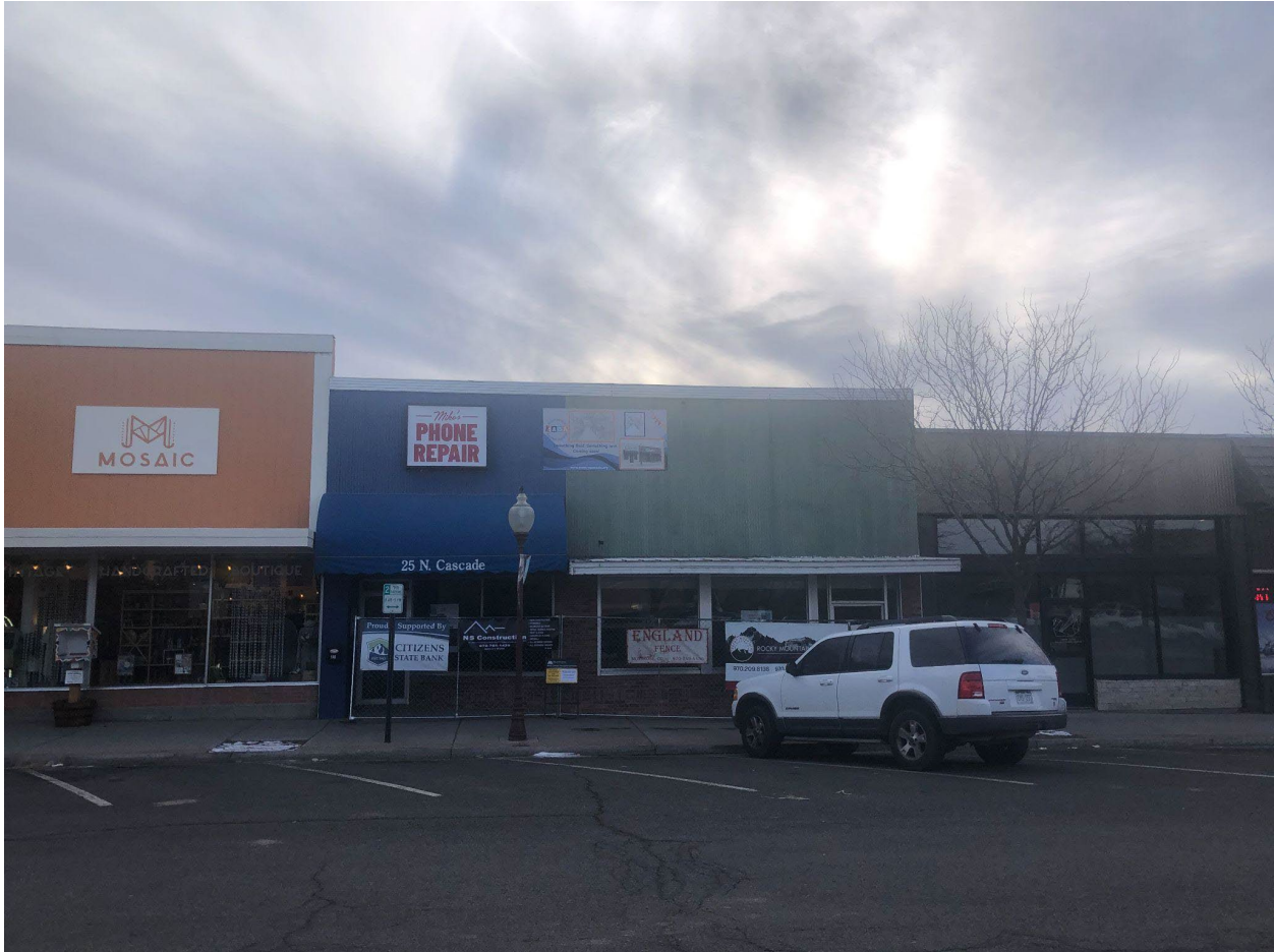
Front facade. Facade has been heavily altered to post-World War II commercial construction. Flat roof with vertical band of metal at roofline. Vertical metal siding above projecting metal awning. Entrances have glazed metal frame doors surmounted by transoms.
