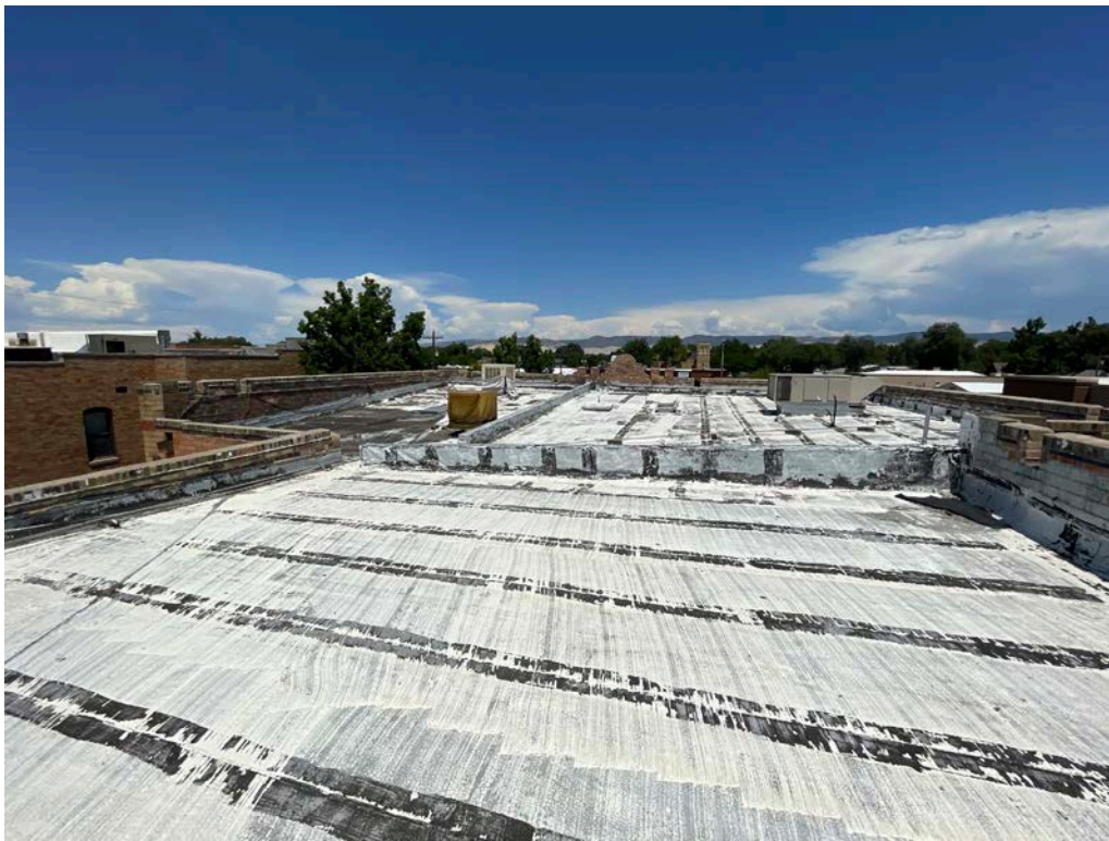
Photo 38: Roof, view east. Approximate midpoint of building.
