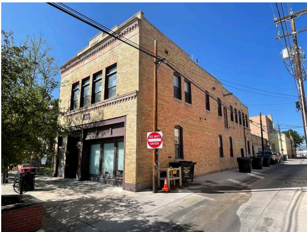
Photo 81: Annex northeast corner and corresponding elevations
