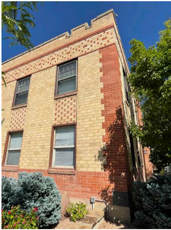
Photo 8: Southeast corner, exterior elevation.
