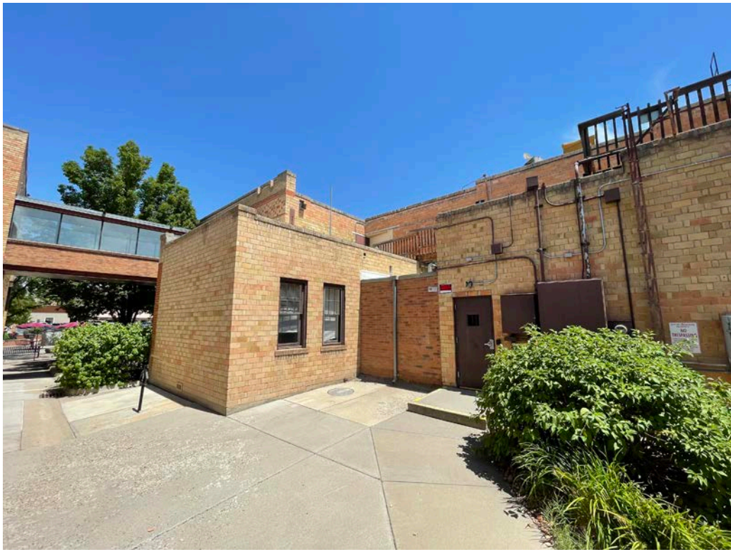
Photo 50: North exterior elevation.
