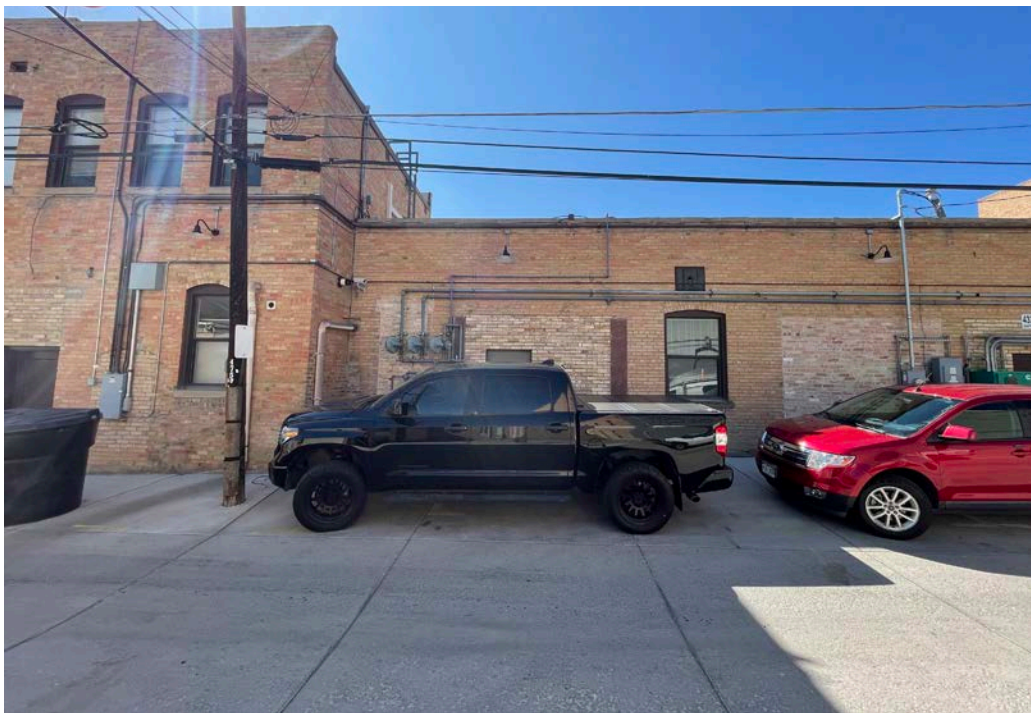
Photo 83: Annex north elevation, center section, step down from 2 story to 2 story.
