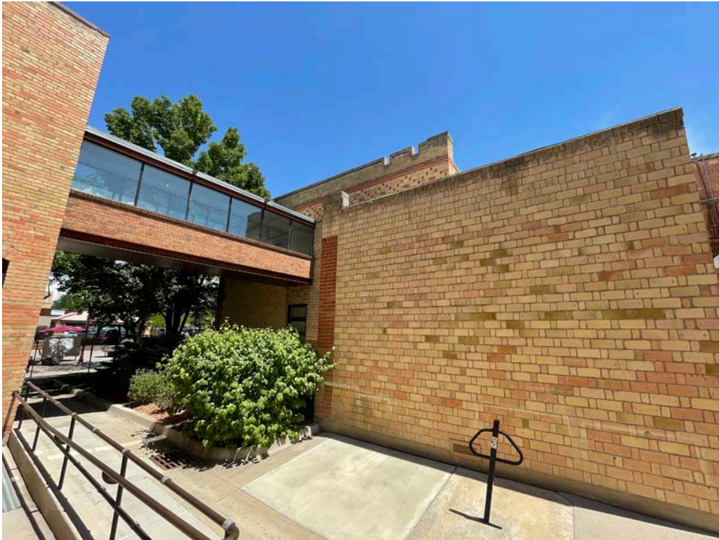
Photo 47: North exterior elevation.
