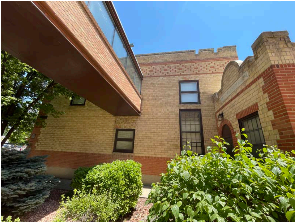
Photo 46: North exterior elevation.
