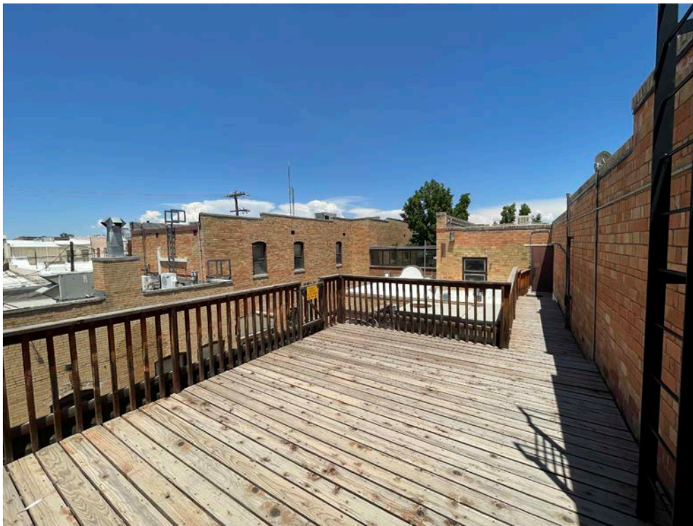
Photo 32: View east, northeast, second floor roof deck.
