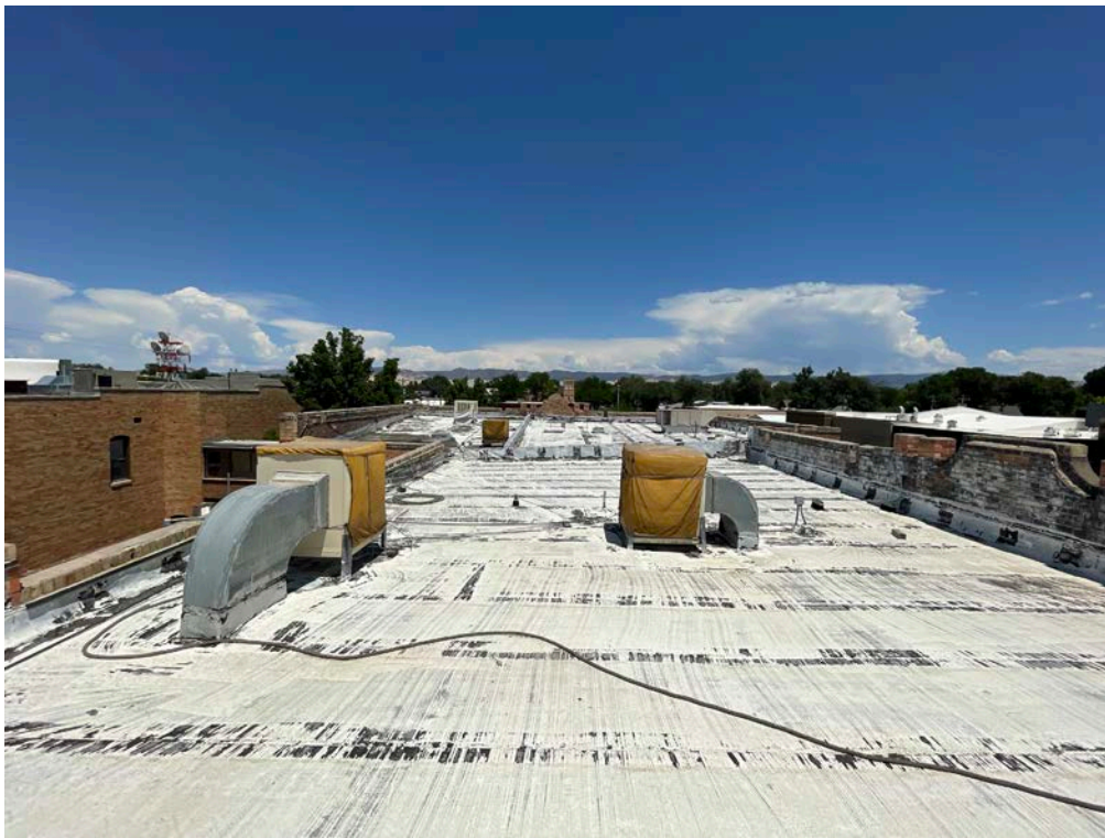
Photo 36: Roof. View east.
