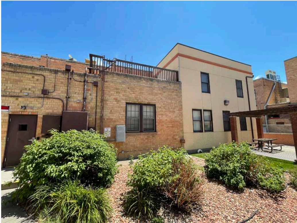
Photo 51: North exterior elevation.
