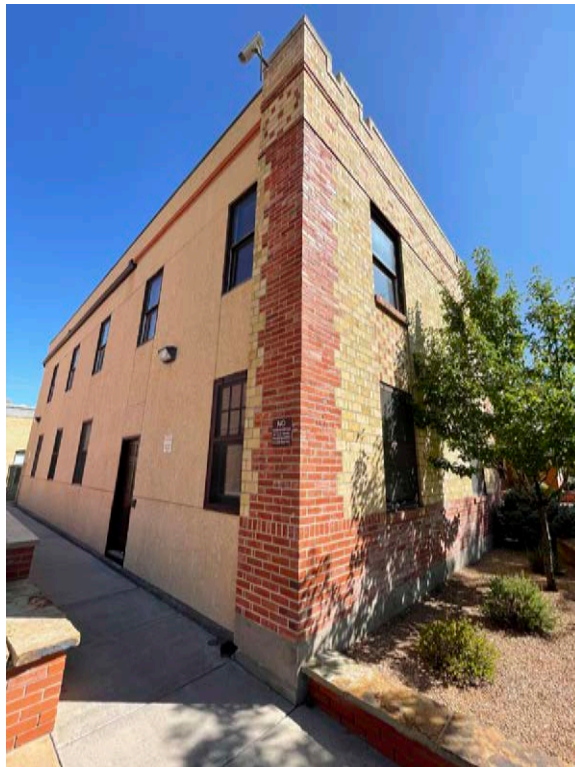
Photo 5: Southwest corner, exterior elevation.
