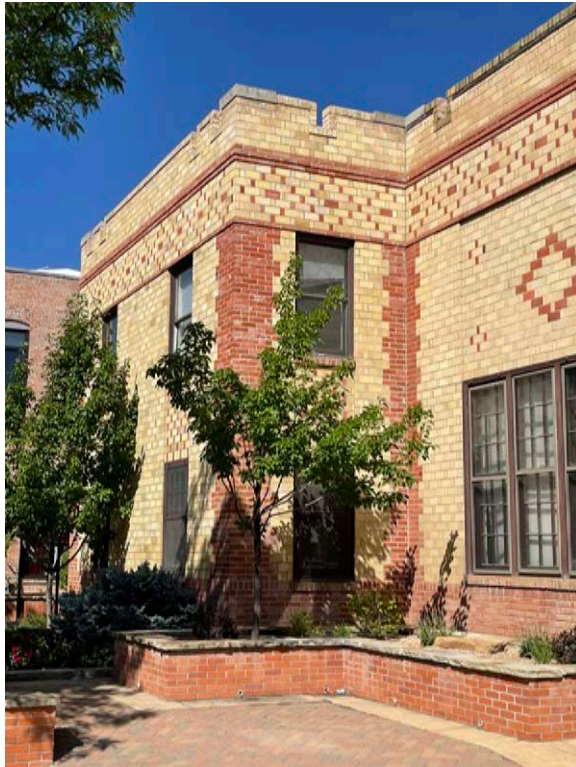
Photo 9: View to the northwest, of southern elevation, west wing.
