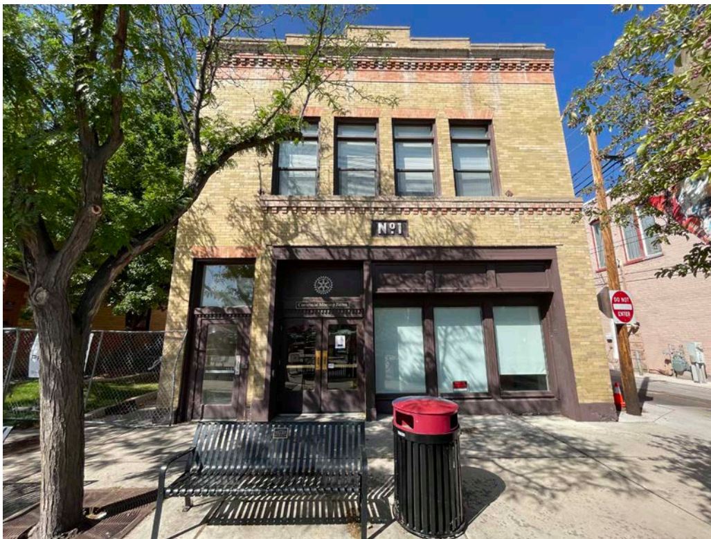
Photo 80: Annex East Elevation
