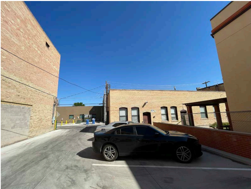
Photo 85: Annex south elevation, west end of building at alley. Montrose City IT Area.
