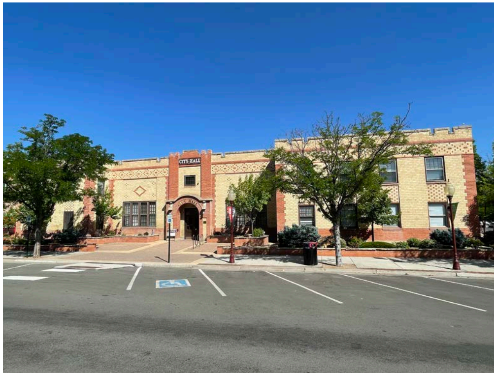
Photo 1: South exterior elevation.
