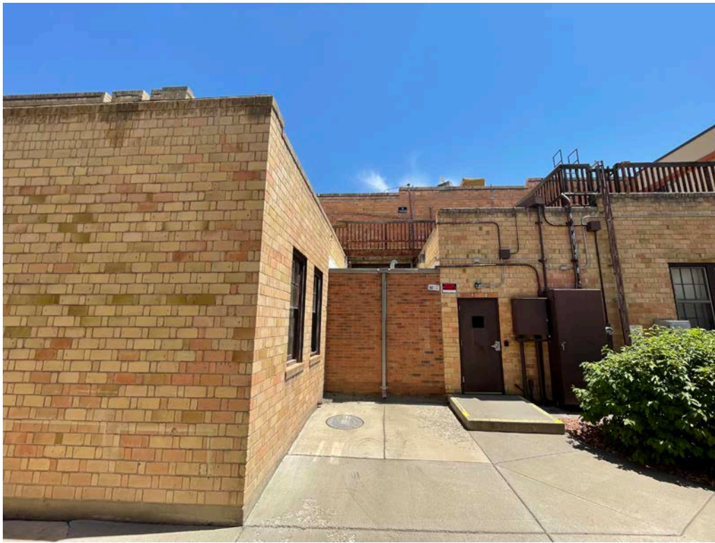
Photo 48: North exterior elevation.
