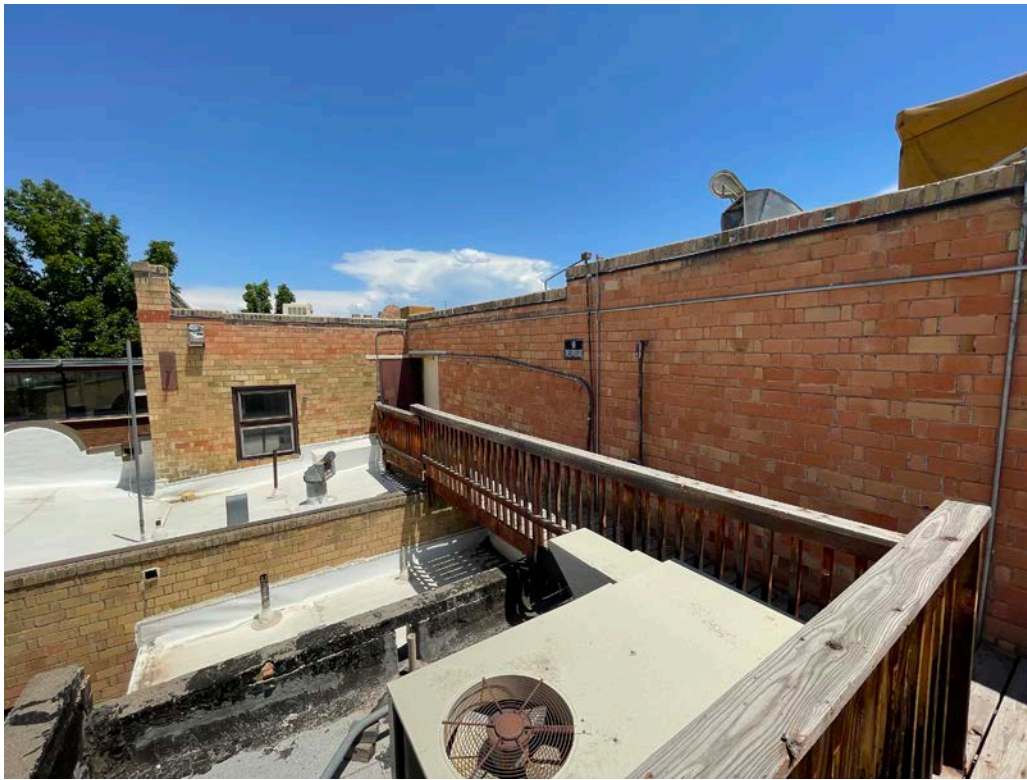
Photo 34: View east, southeast, second floor roof deck.
