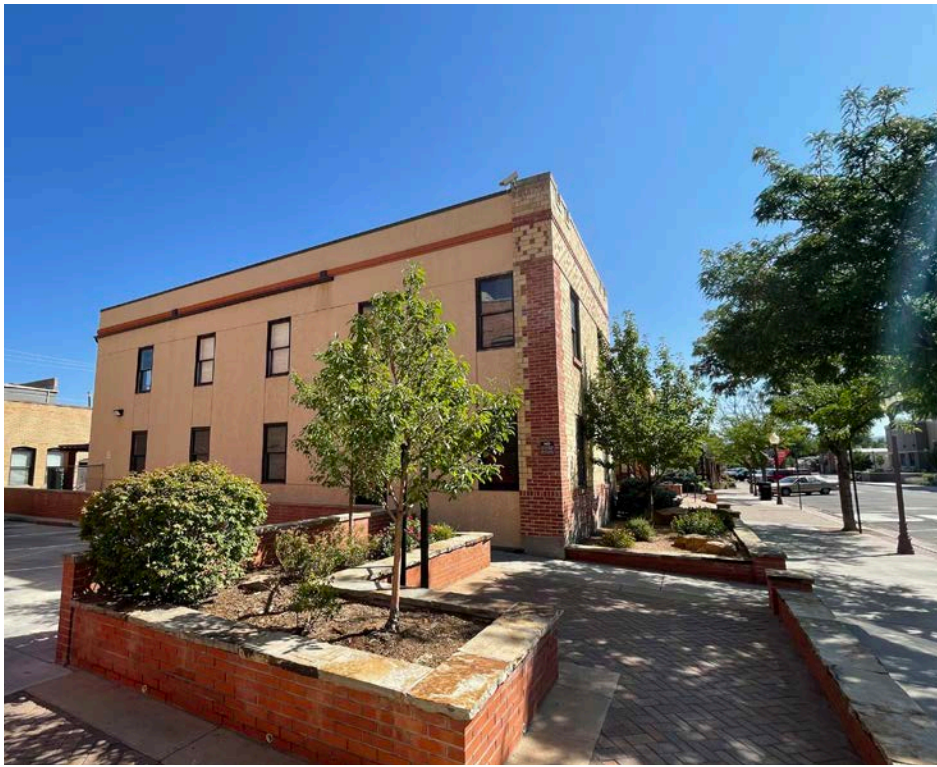
Photo 4: East exterior elevation.
