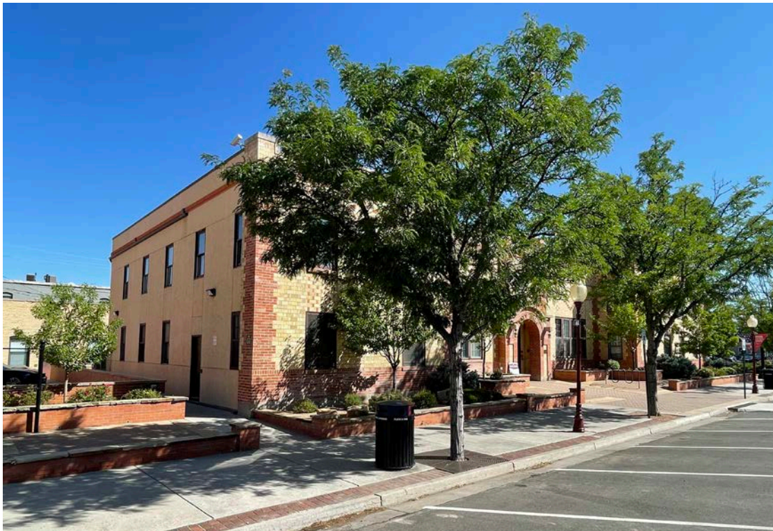
Photo 3: Southwest corner, exterior elevation.
