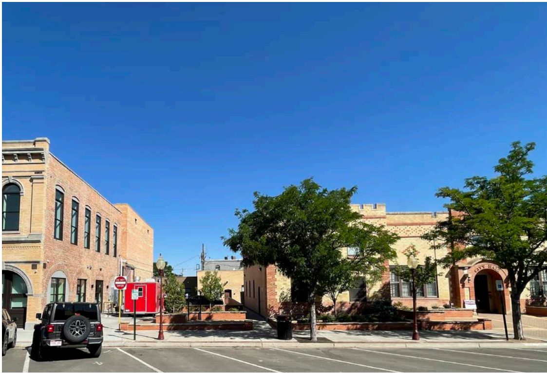
Photo 2: South exterior elevation. West end of building.
