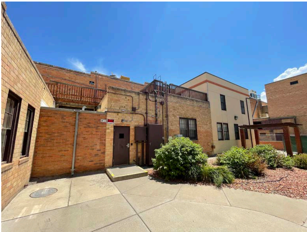
Photo 49: North exterior elevation.
