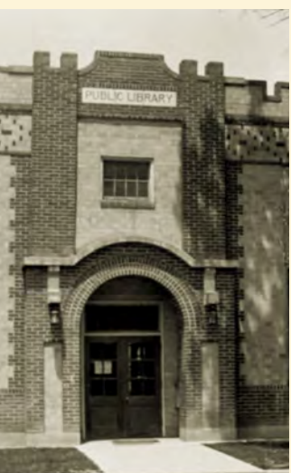
★ National Register of Historic Places * Local Register of Historic Places
