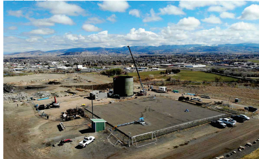
Photo of one of the City's water facilities
