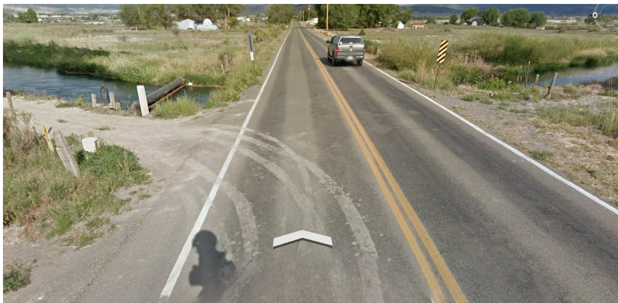
Photo 1: Existing Ogden Road Culvert Crossing
