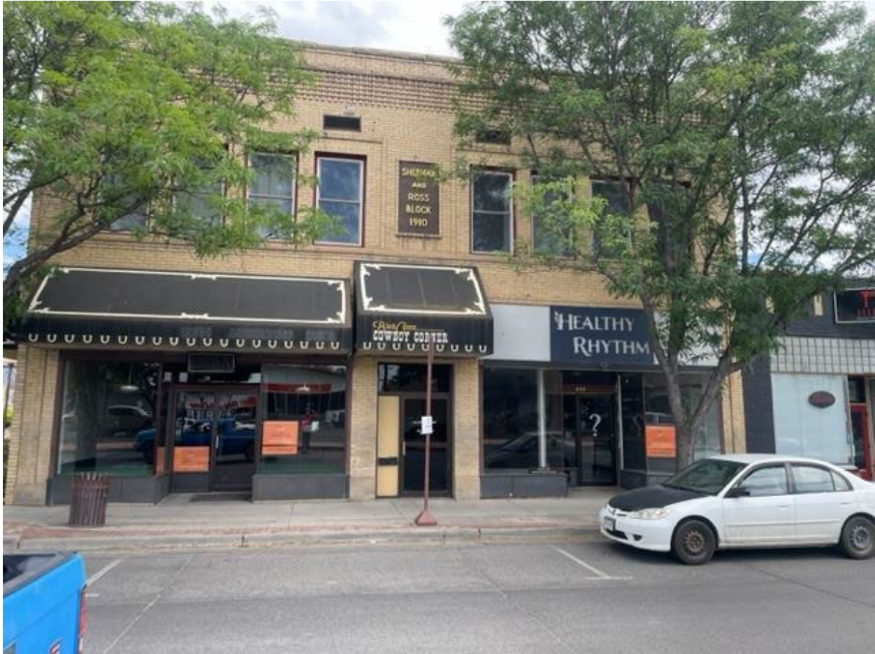
Front facade. Yellow brick and cornice of decorative brickwork, with series of rectangular vents under cornice. The second story is divided into two bays with four double-hung sash windows in each bay enframed with brick. Continuous stone sill course at second story. Between the two bays of the second story is a metal plaque inscribed "Sherman And Ross Block 1910."
