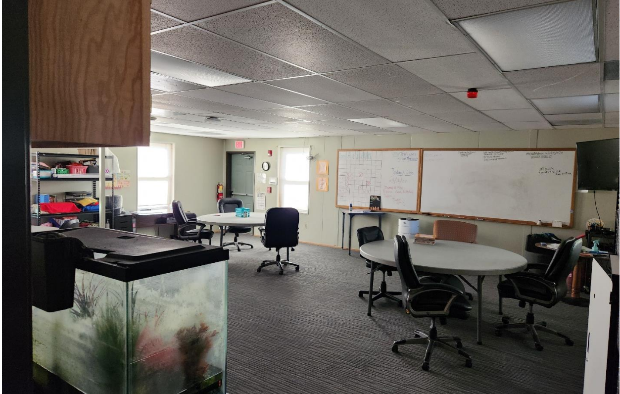
Typical interior finish of existing classroom
