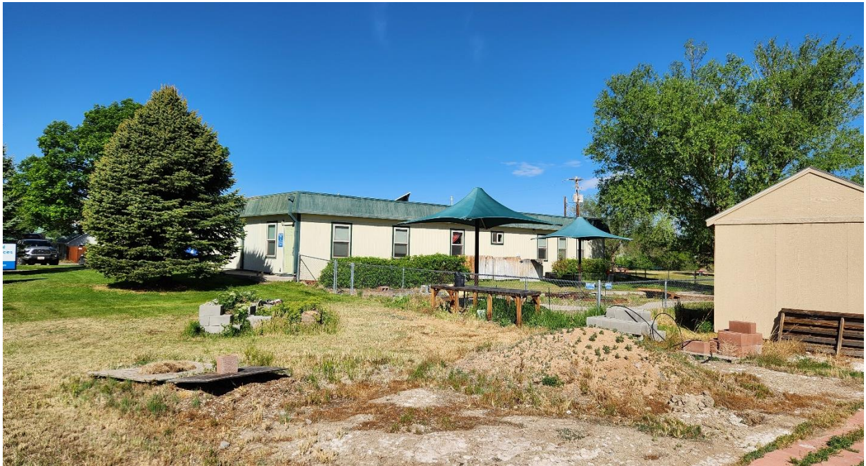
View of property from southeastern property corner
