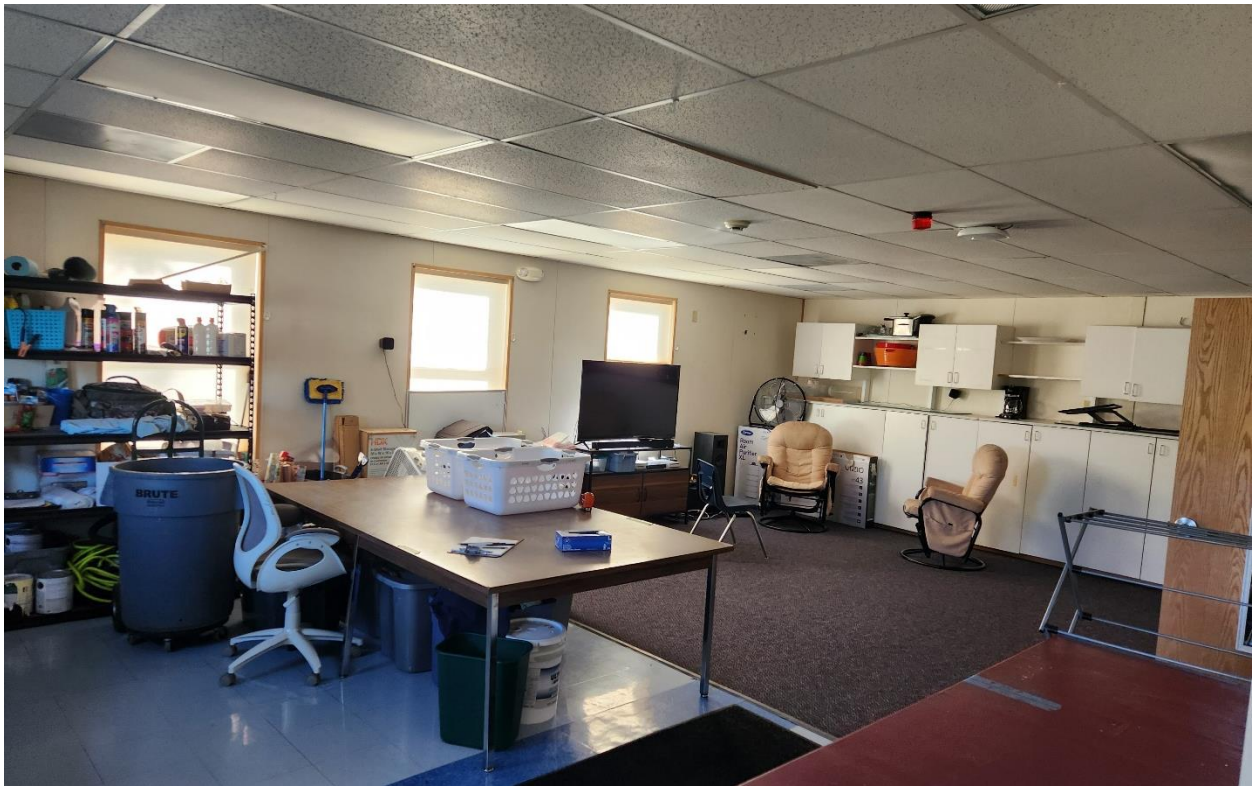
Typical interior finish of existing classroom
