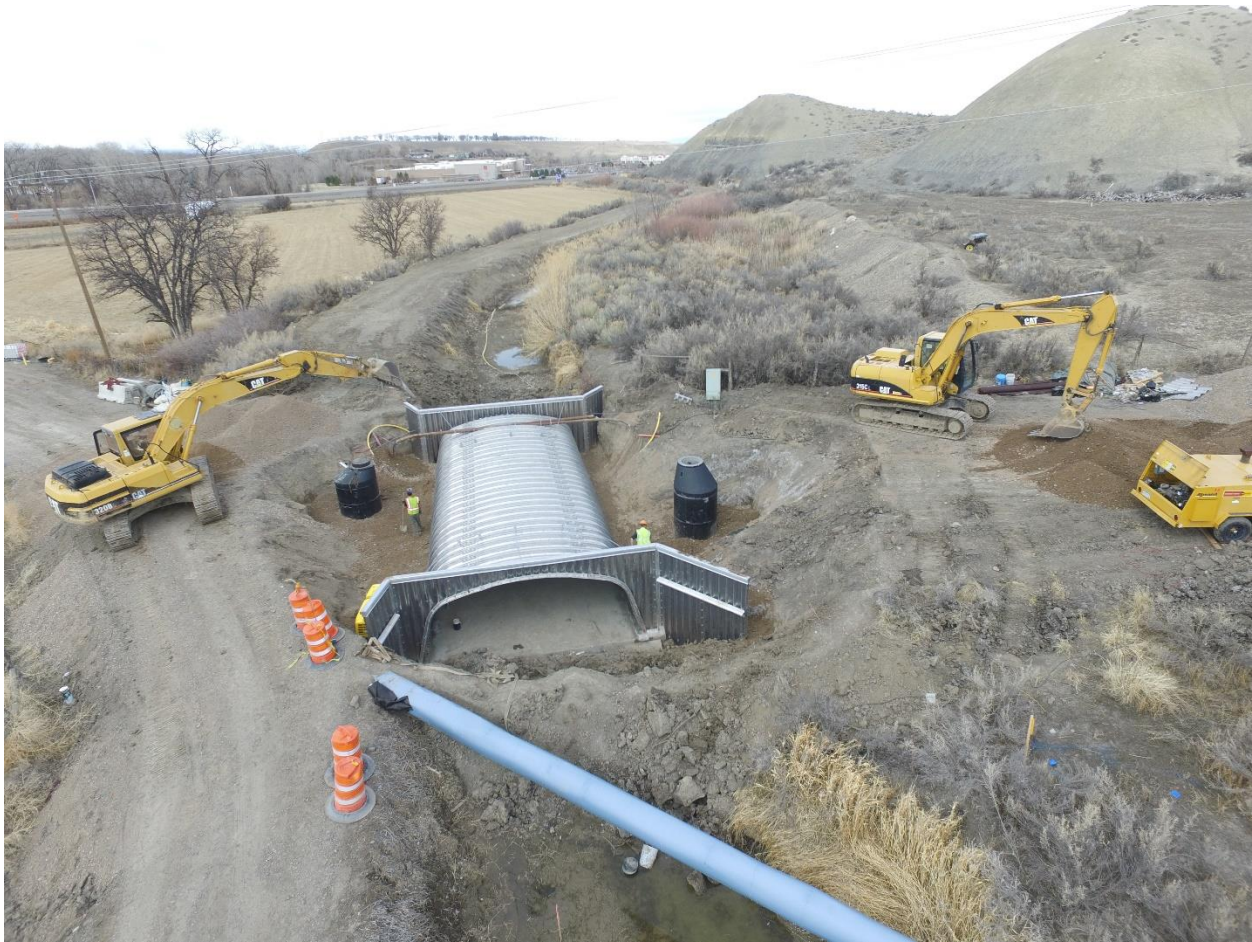
Photo 1: Otter Road Example Project under Construction
