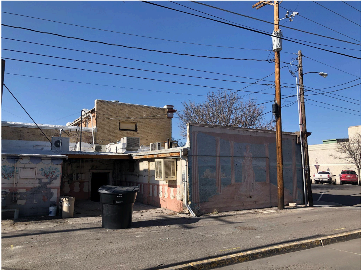
Rear/alley side. The original rear of the two story building can still be seen. The one-story extension is
