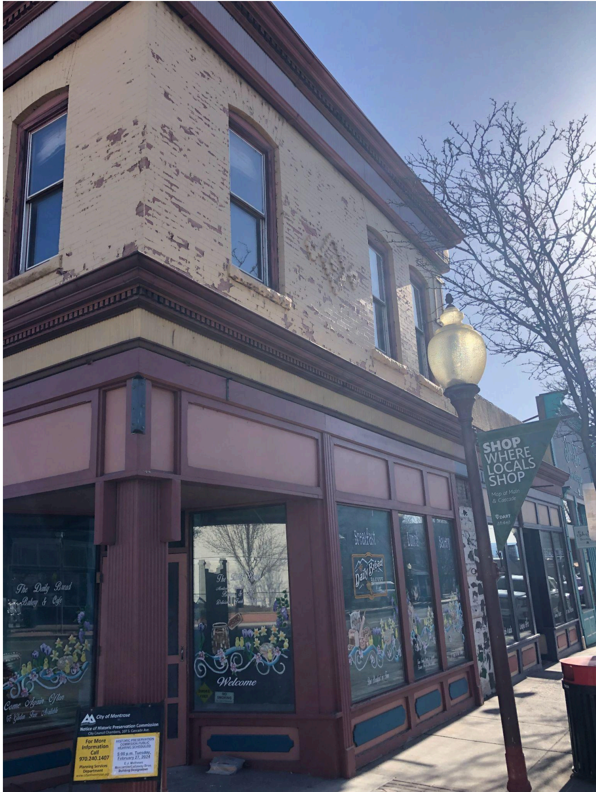
Front/Main St side. Second story windows retain stone sills and arched transoms. First story has been remodeled.
