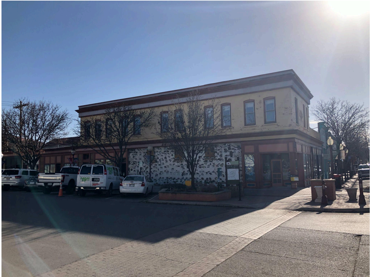
S Cascade Side. Note that the chimneys along the roofline have been removed. Decorative brickwork, secondary cornice with dentils remains extant.
