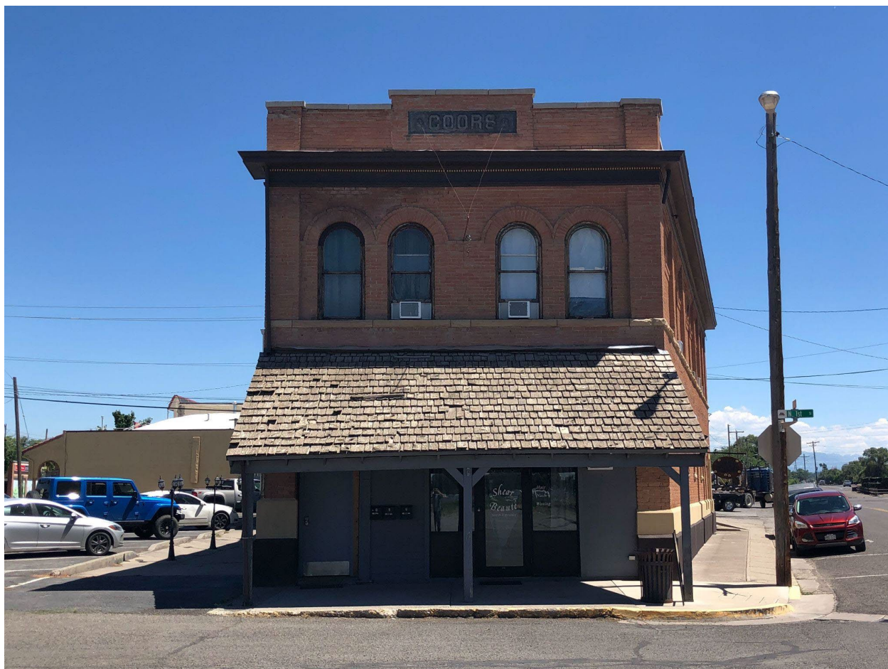
Front facade/North 1st St. Note the central parapet with the metal panel inscribed "COORS." Brick coping along roof slightly projects. The facade has two sets of paired round arched windows and a continuous rock-faced stone sill course. The first story has been altered, including the porch addition.
