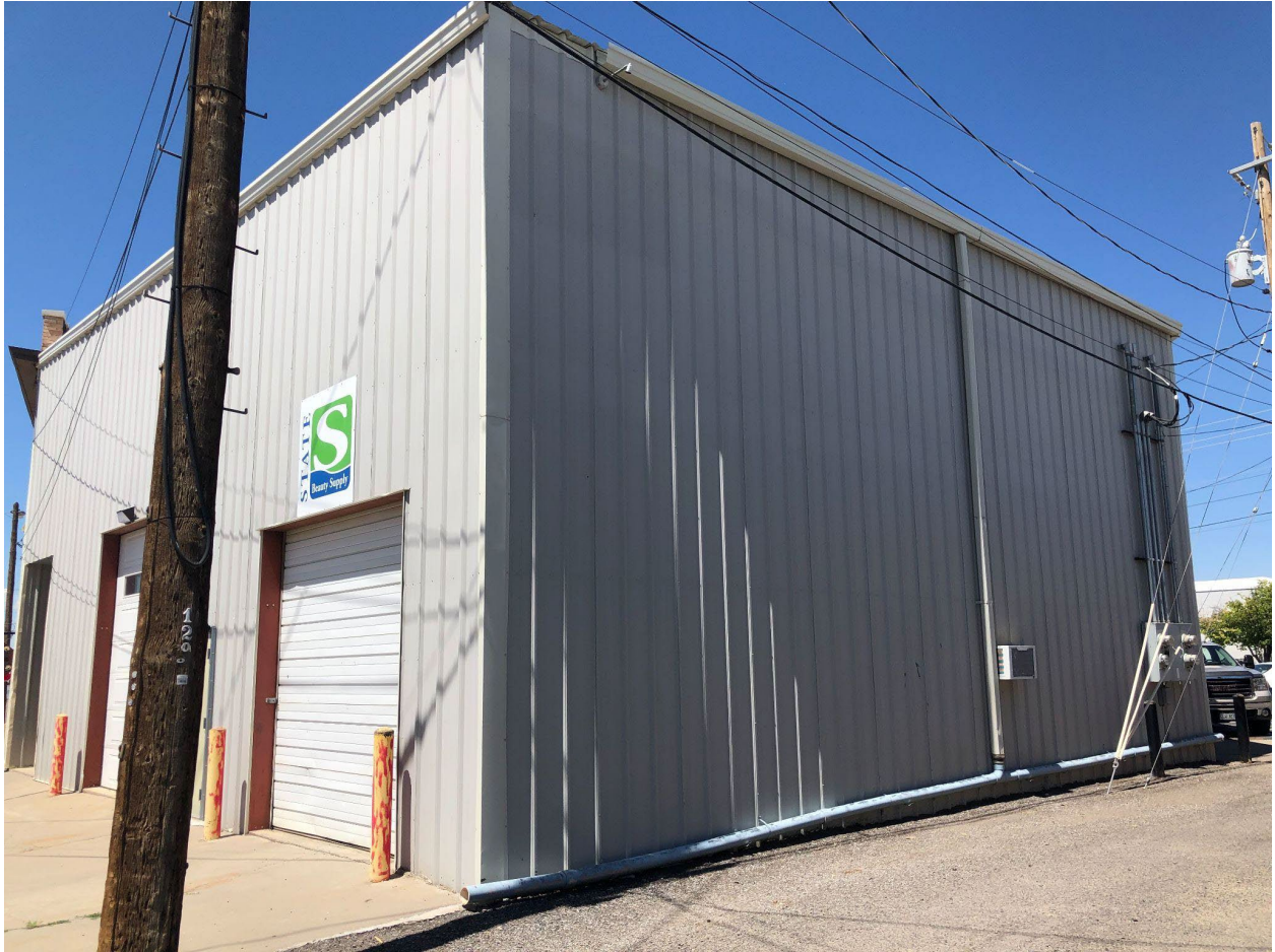
Rear/alley-facing side. This addition has heavily altered the rear of the building, and no notable historical characteristics can be seen.
