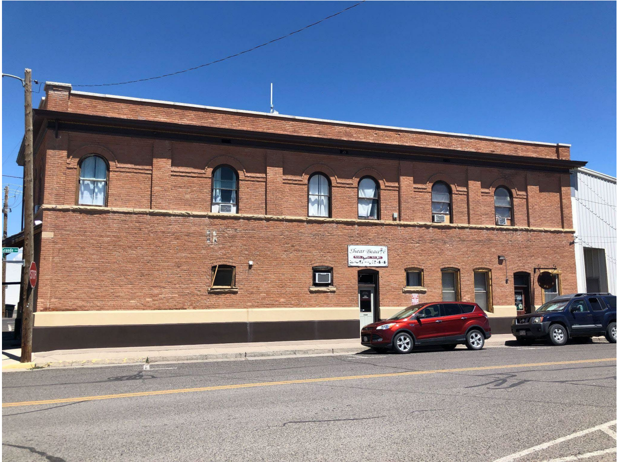
N Rio Grande Ave side. Concrete with beveled top on lower wall. Rock-faced stone sill course continues from the front facade. Cornice and corbelled brick above second story windows. Slightly projecting piers define five bays on wall.
