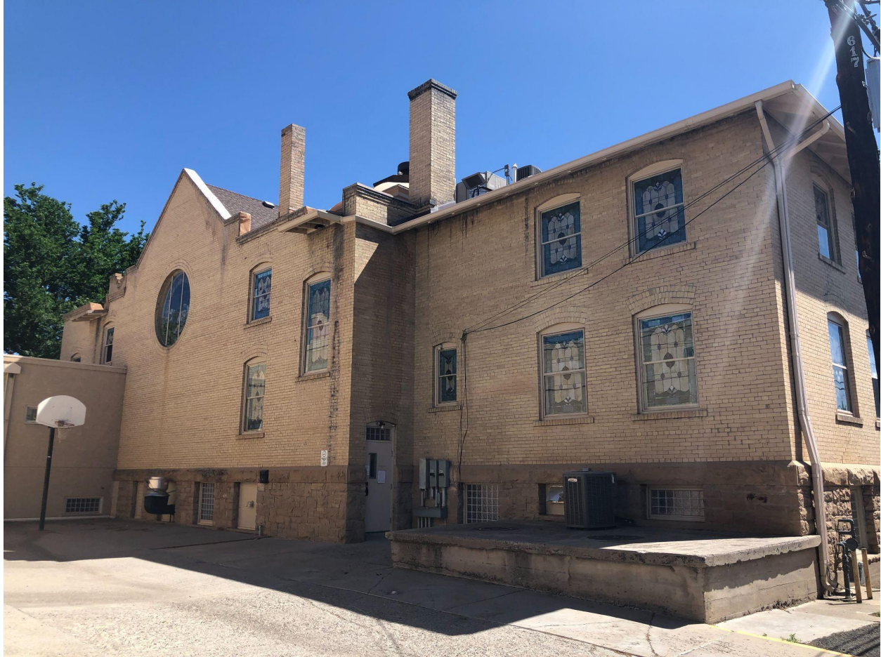
Rear (northeast) side
