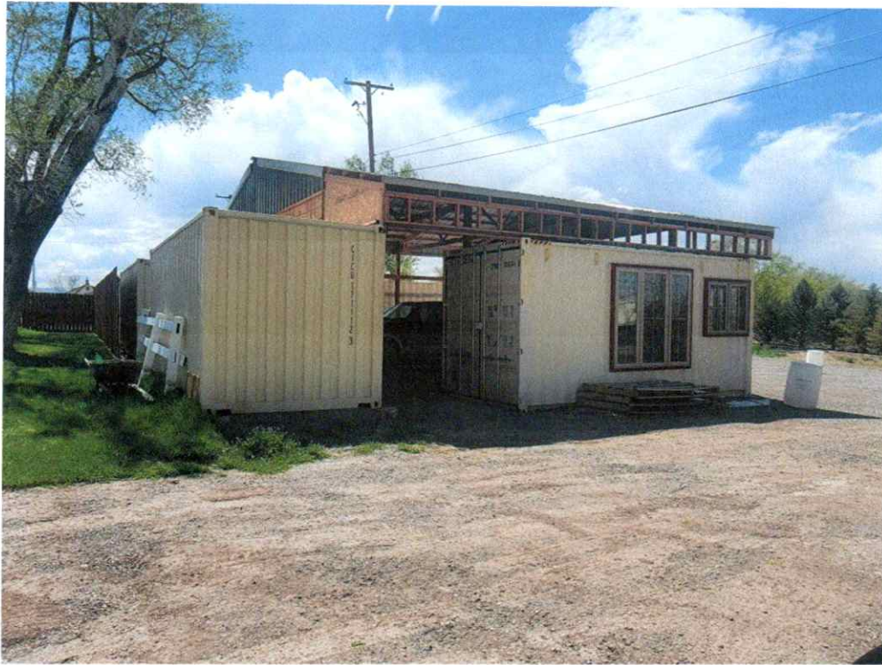
Connex Unit Barn
