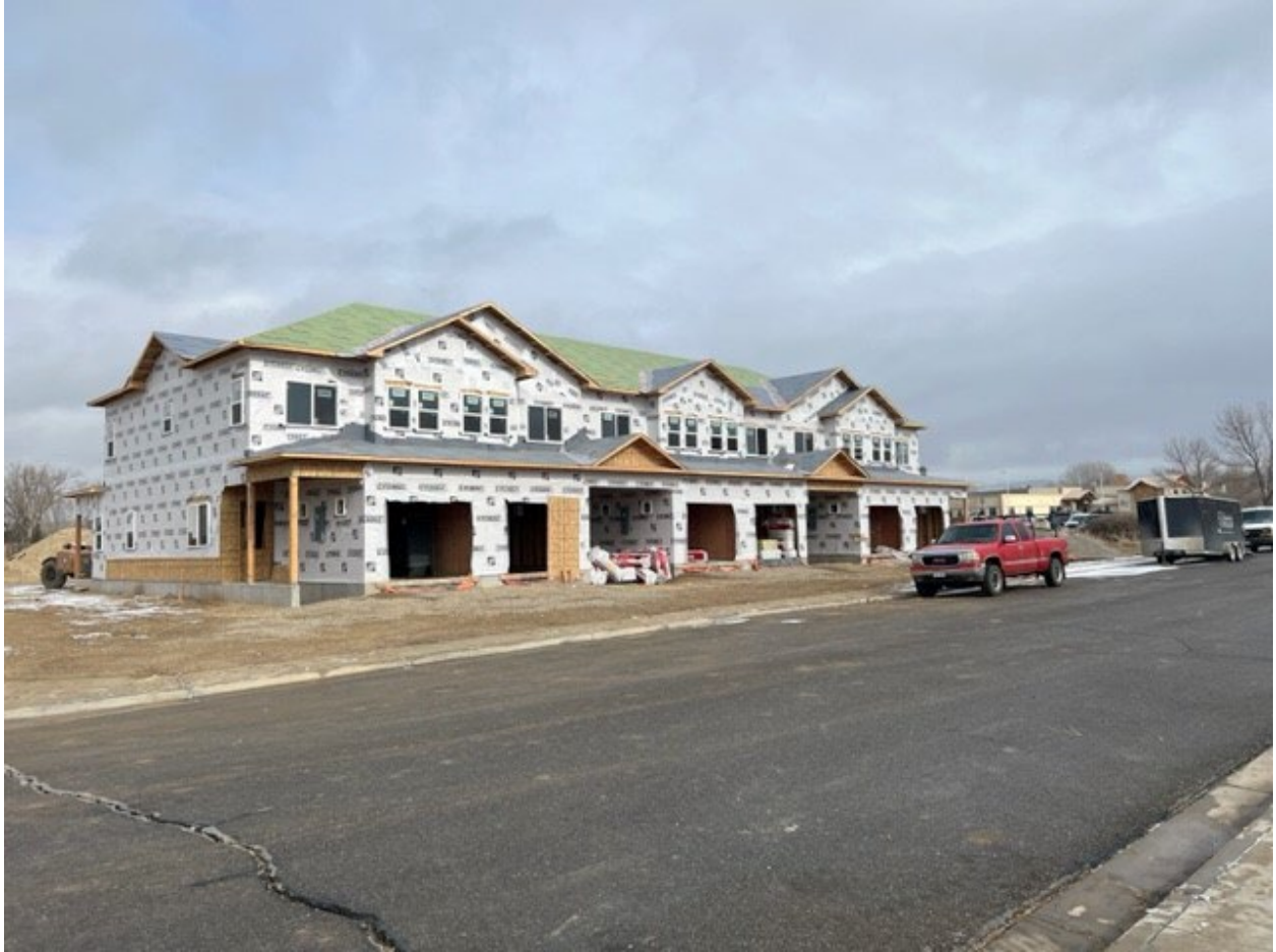
6-plex under construction on Lot 5
