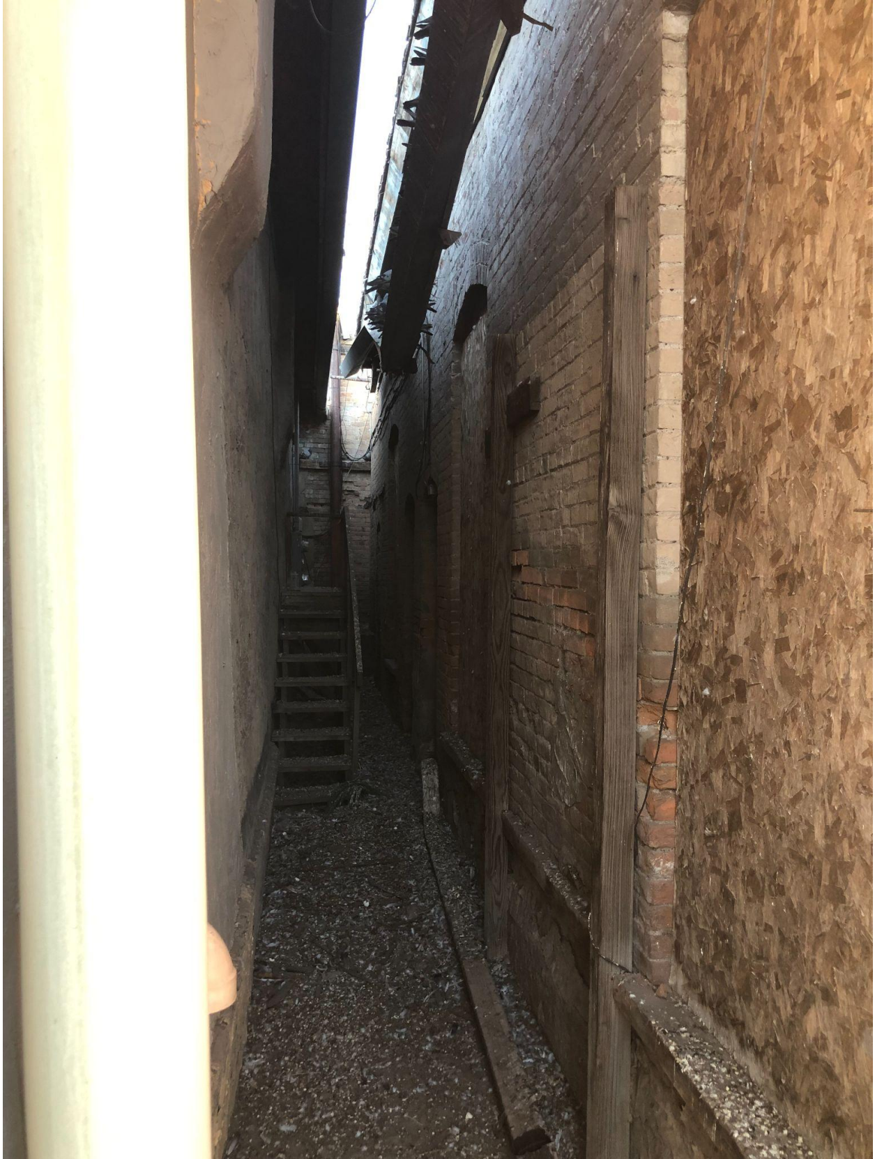
Northwest side. The brick exterior can still be seen on this side. Window openings have retained their shape.
