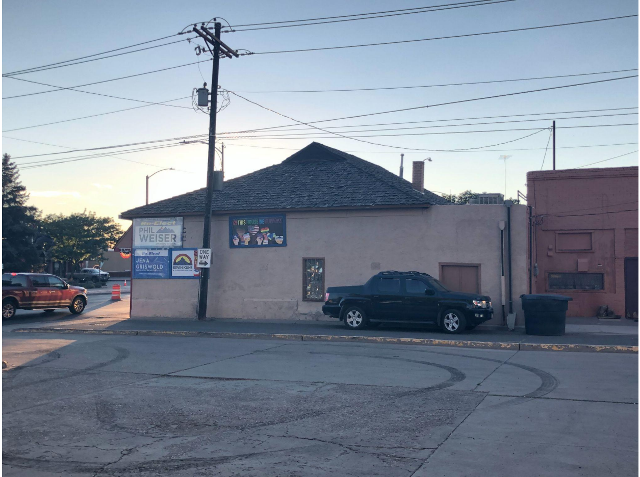
Southeast side. Note the gable-on-hip roof. The small addition on the northeast side was added sometime between 1899 and 1904. A window and possible entrance on the left of this picture has been covered.
