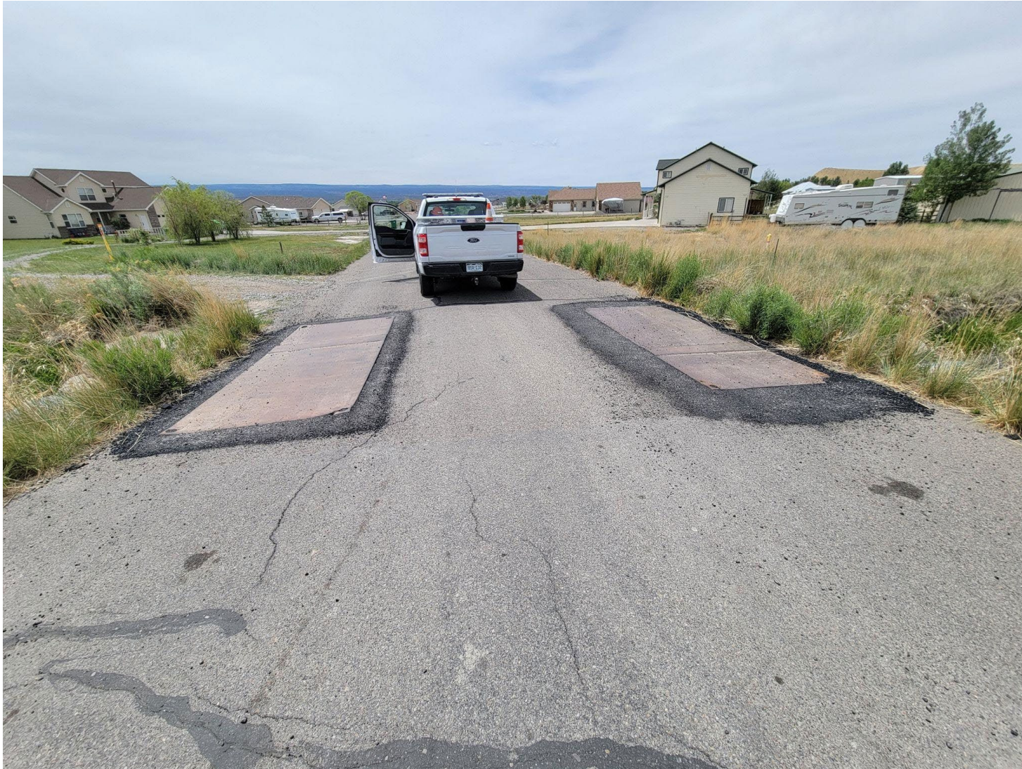
Photo 5: Overland Drive Temp Repair
