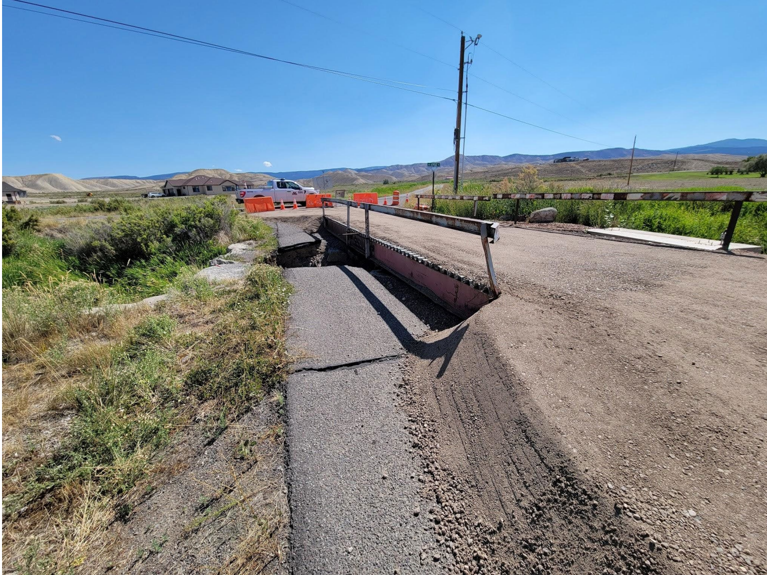
Photo 6: Open Field Drive Temp. Bridge
