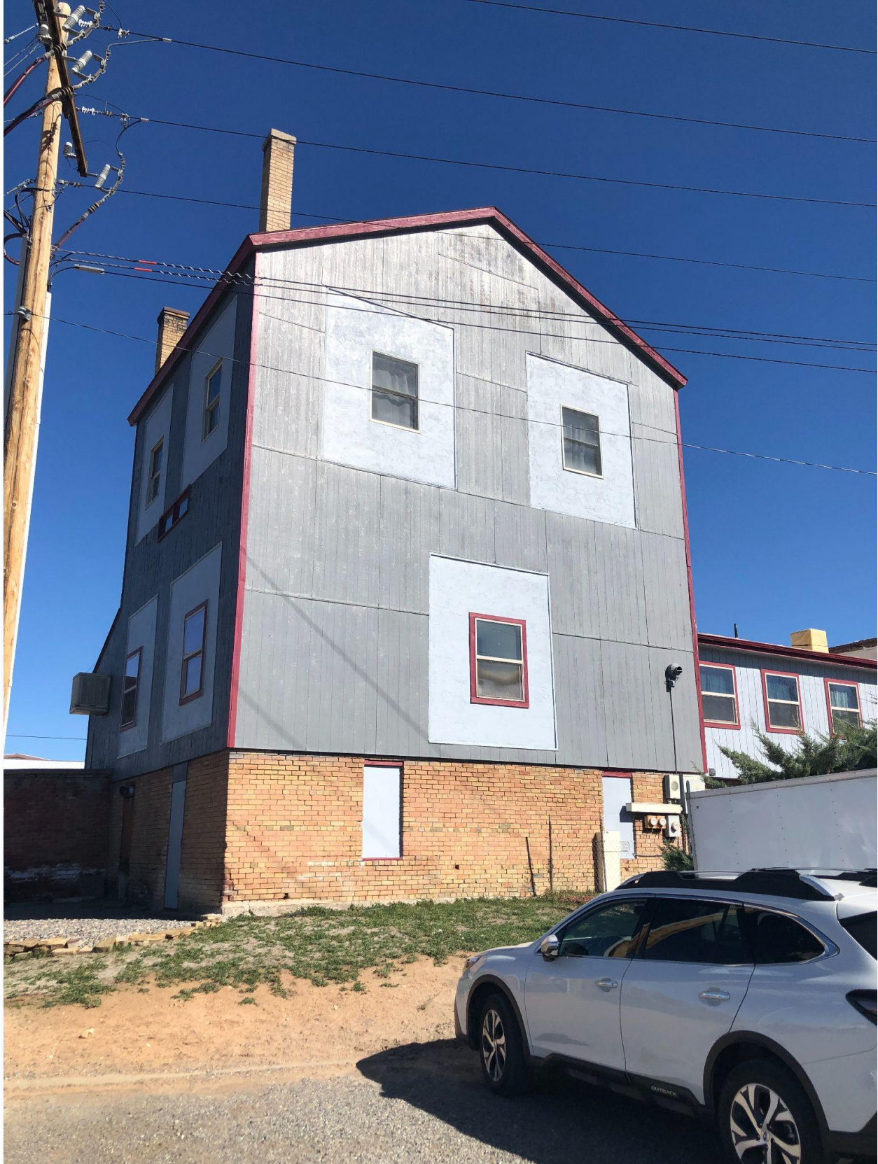
East side. Note the brick basement, as well as the brick chimneys and gable roof.
