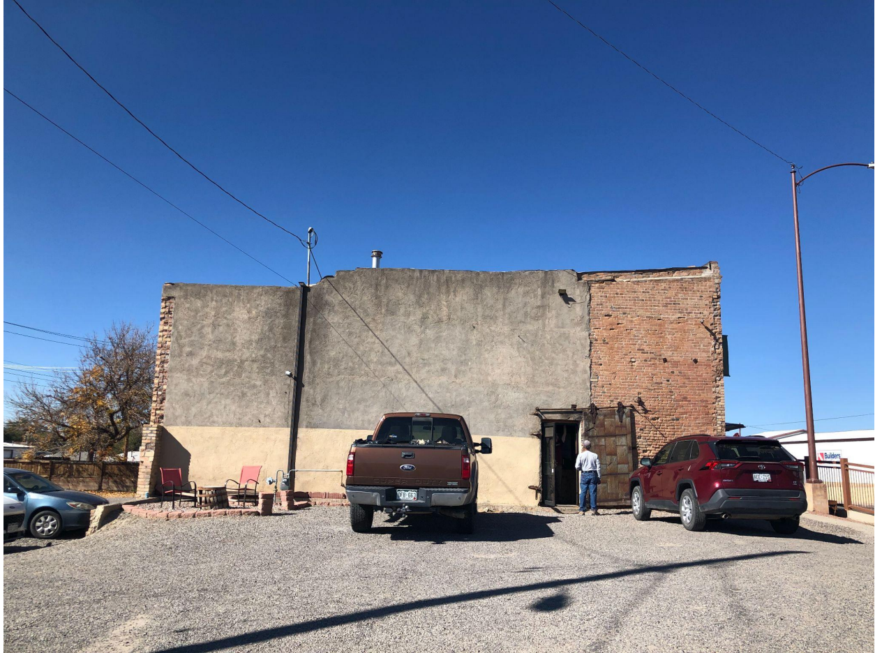
South side. This side would have been where the three horizontal boilers once stood. This has been demolished, but remnants of the brick structure still remain on the sides.
