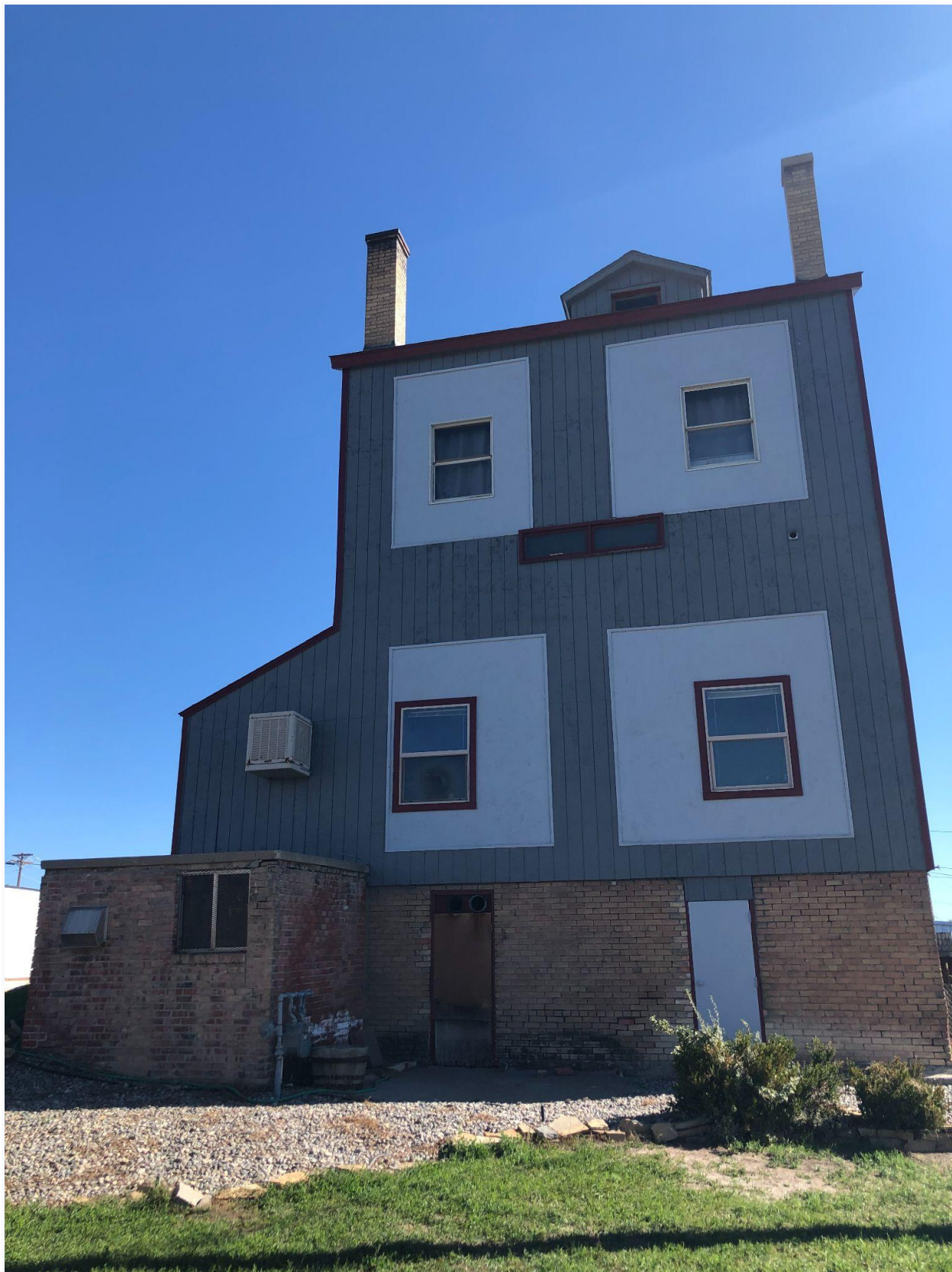
North side. The brick basement can be seen on this side, as well as the brick chimney, and the dormer window with is mirrored from the south side.
