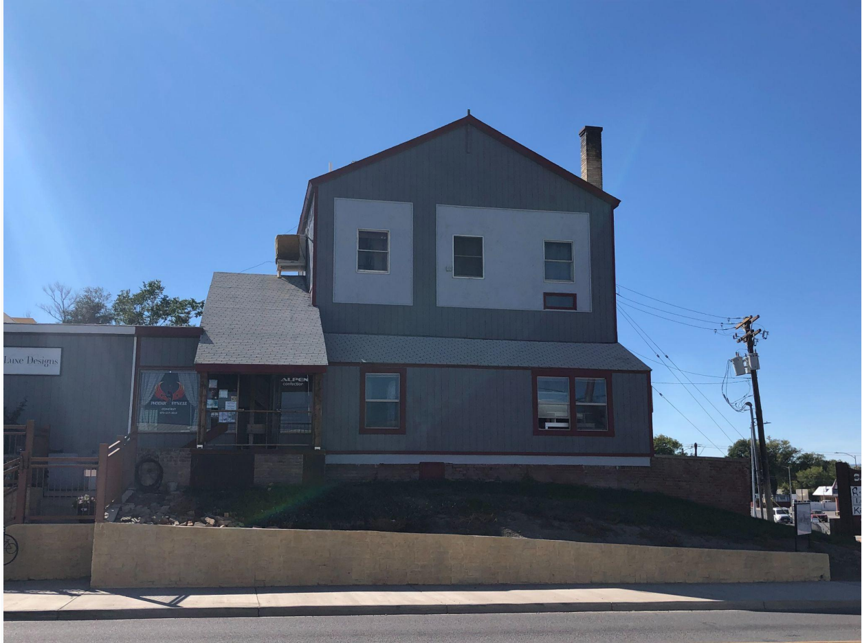
East facade. The shed roof projection has been extended to the entire facade.
