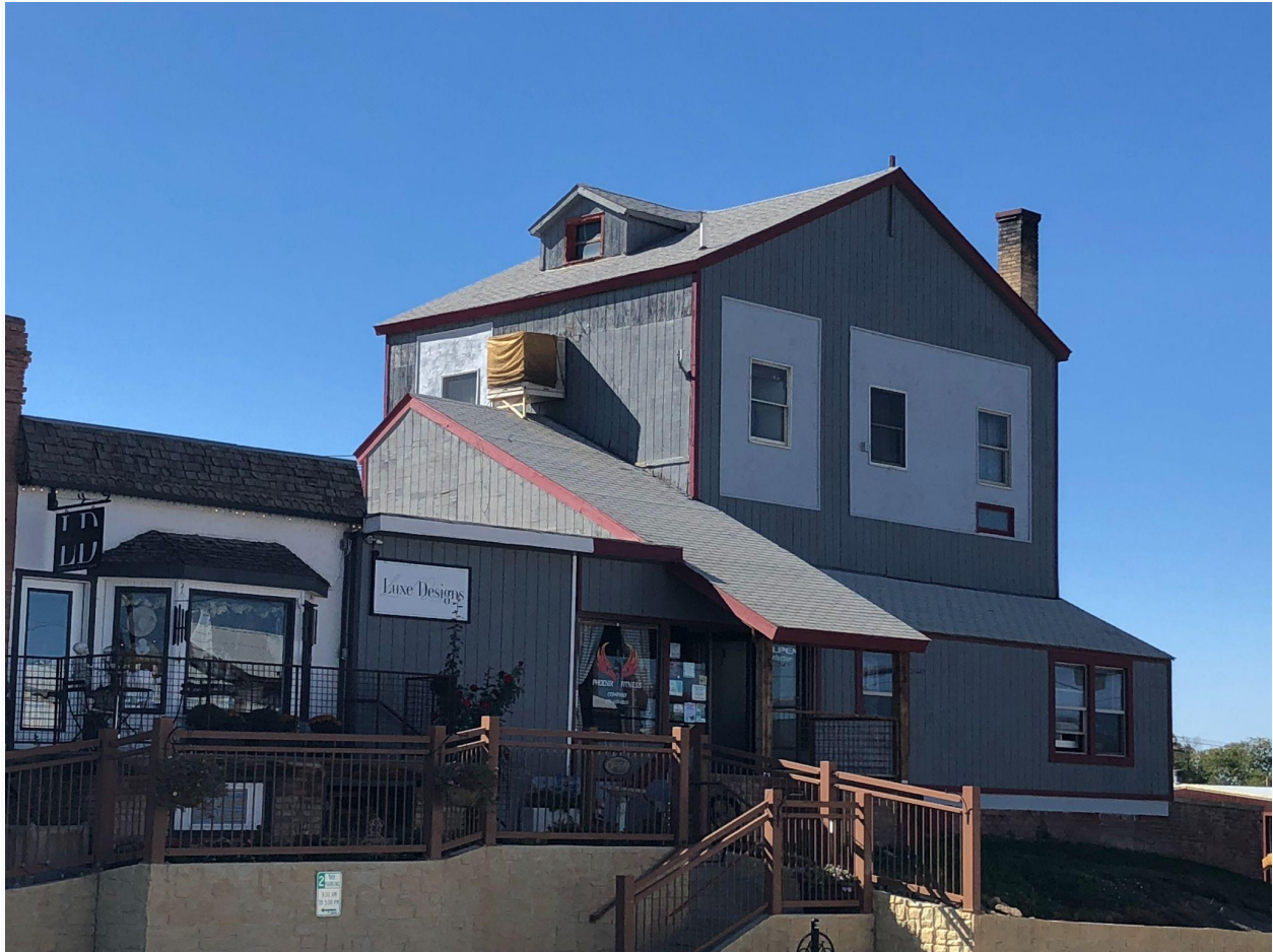
South side. Note the dormer window on the second floor. The connection to the Montrose Electric Light & Power Co. is a recent addition from 1974.
