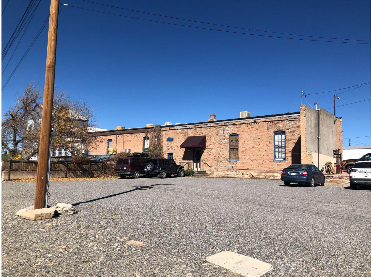
West side. Note the arched brick above the windows. The middle window has been modified and partially covered with brick.
